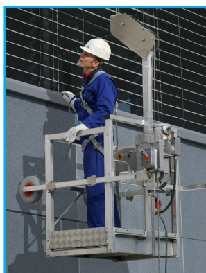
Work seat during repair work.
