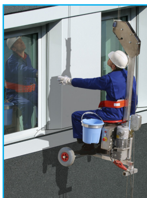
Work basket for assembly work
